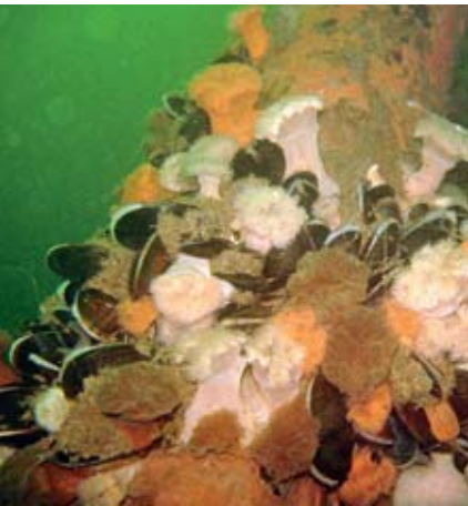
Fig. 25 Marine growth on foundation. Photo: Sebastian Fuhrmann
