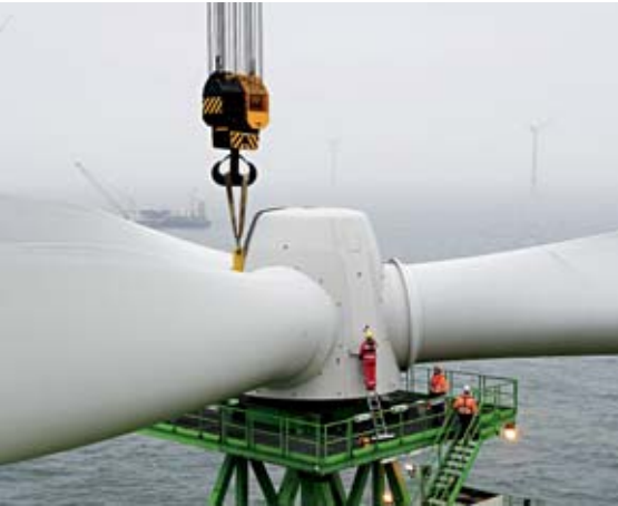
Fig. 3 Erection of a REpower wind turbine Photo: DOTI 2009
