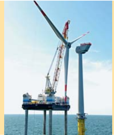
Fig. 7 Raising the rotor blade star Photo: DOTI 2009
