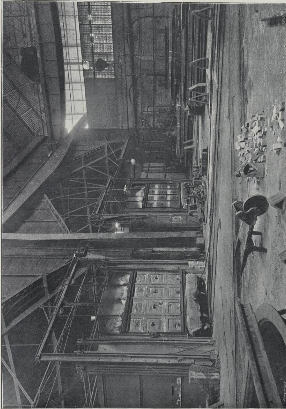
FURNACES OF THE BOGIE TYPE FOR THE CARBURISING OF ARMOUR.
