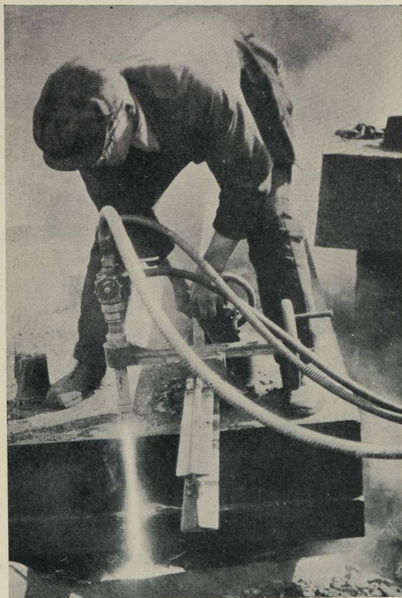
FIG. 14.—RAY CUTTING STEEL PLATES 14\frac{3}{4} IN. THICK WITH OXYGEN.
