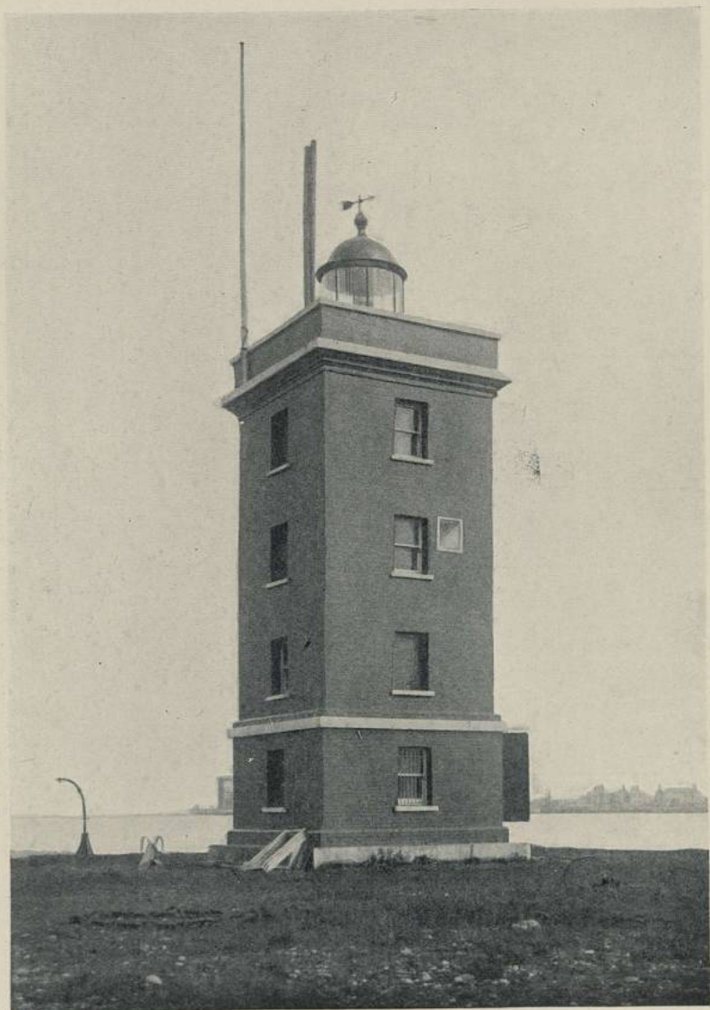
FIG. 92B.—BREAKWATER LIGHTHOUSE, DUBLIN. (Showing small white window for entry of a beam of light. See p. 120.)
