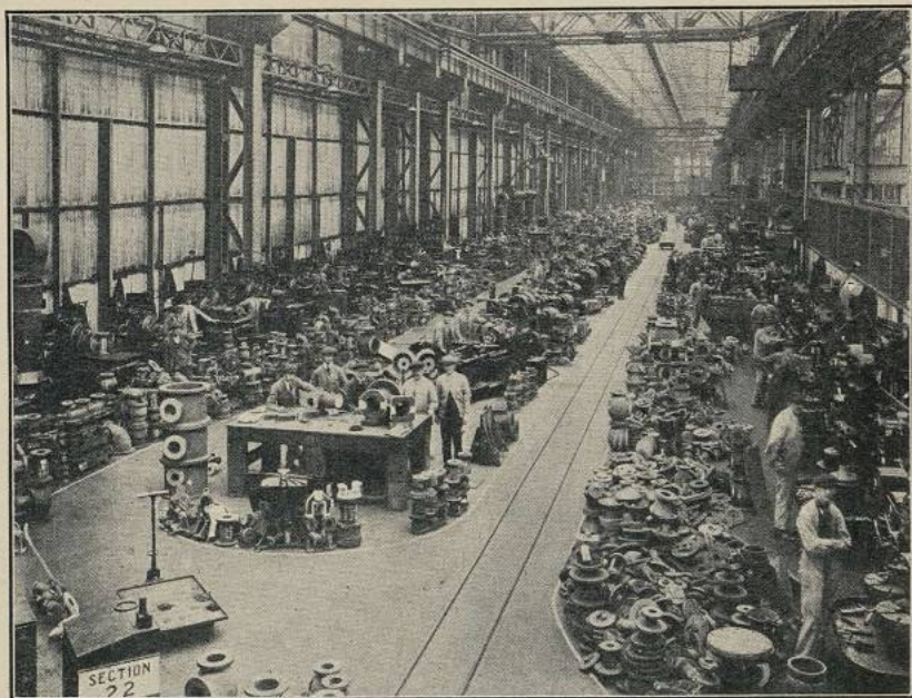
FIG. 10.—VALVE SHOP, QUEEN'S ISLAND, BELFAST. (P. 19.)
