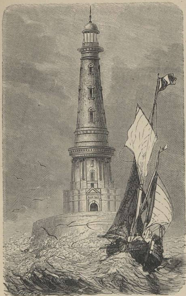
PRESENT LIGHTHOUSE OF CORDOUAN.
